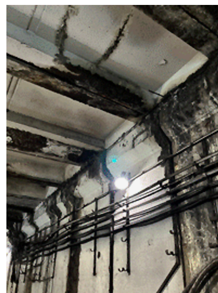
Fig. 3. Leaching and destruction of the concrete structure of the roof slab due to erosion of the waterproofing barrier
