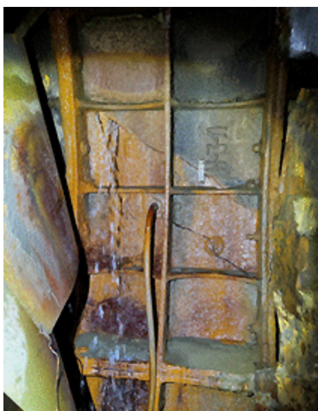
Fig. 1. Leaching and wet spots at the inter-ring and inter-block joints of the tubing lining, active leakage. Crack in the back of the tubing
