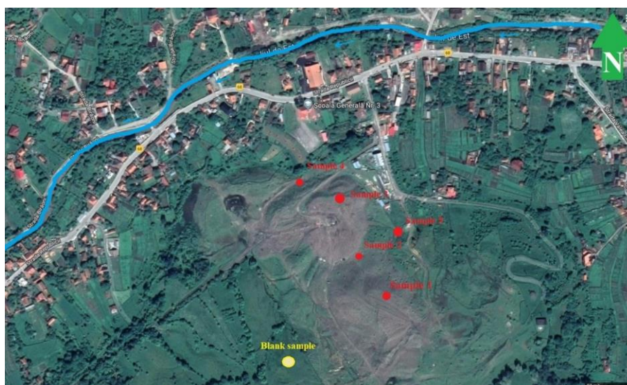
Fig. 4. Lonea 1 tailings storage facility
