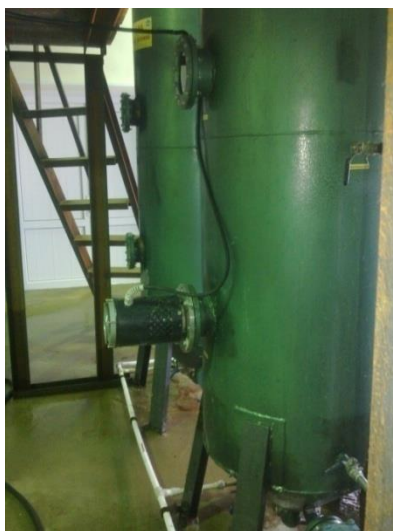
Fig. 3. Installation of the ultrasonic unit on the SNK-640 ion exchange column
